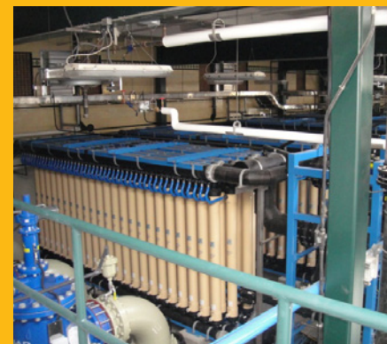
Membrane Rack #1. Each rack contains 94 modules and the City has 4 racks.
